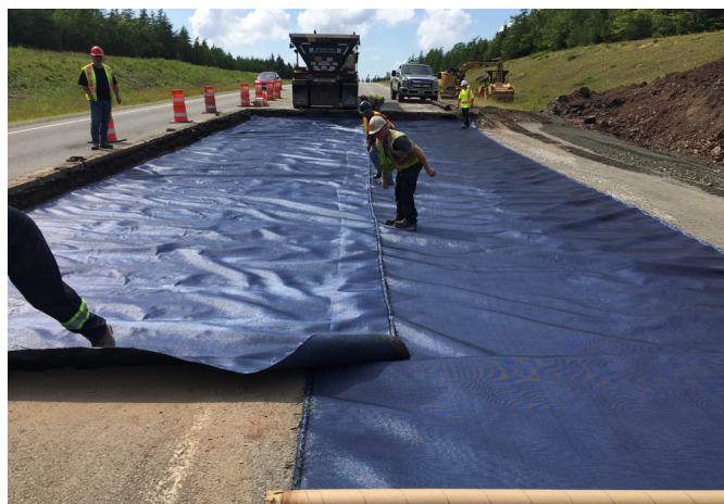
Figure 7: Extending the geosynthetic reinforcement up a vertical face
