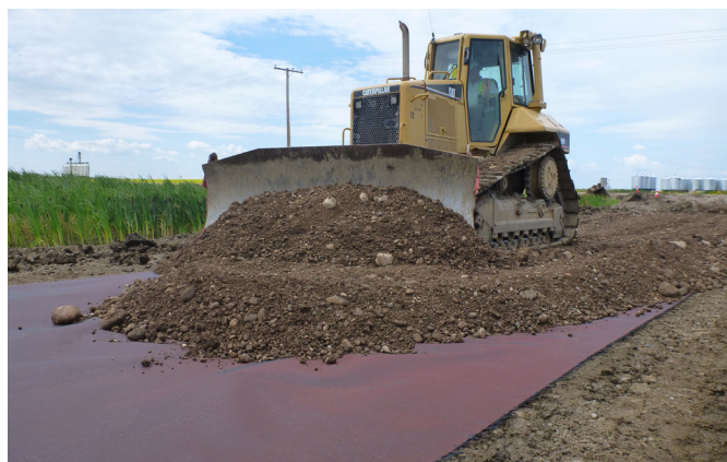
Figure 4: Spreading aggregate over geosynthetic
