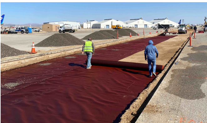
Figure 2: Geosynthetic deployment
