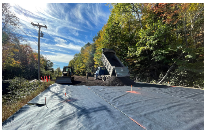
Figure 3: End dumping aggregate
