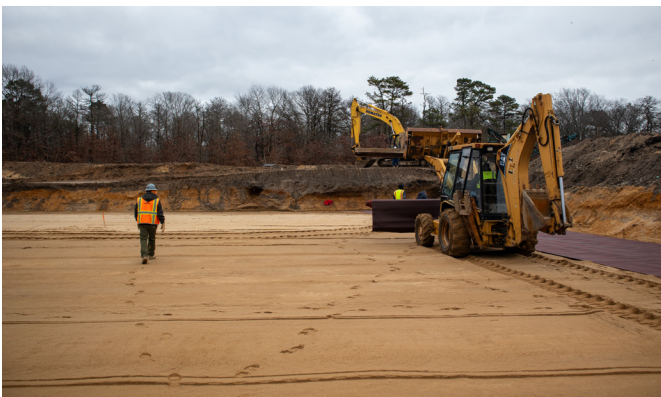
Figure 1: Subgrade preparation
