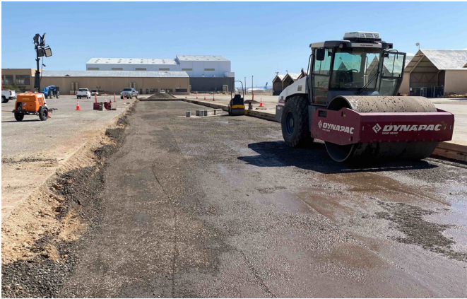
Figure 5: Smooth drum roller
