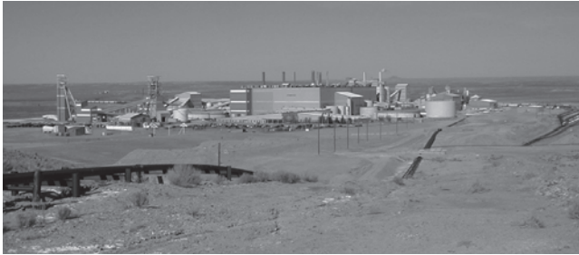
Figure 1 Above-Ground Installation of PE Pipe in a Wyoming Mining Operation
