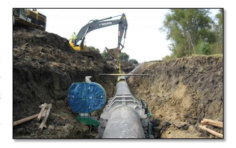
Performance Pipe products can also be connected mechanically when fusion cannot be done due to constructability limitations. Please refer to Performance Pipe's *Field Handbook* for more information. Flange adapters with metal back-up rings, mechanical joint adapters, compression couplings and other means are available for joining PE pipe. More information can be found on *PE Flange Adapter* PP 811-TN and *MJ Adapter Connections* PP 812-TN online at *www.performancepipe.com*.
