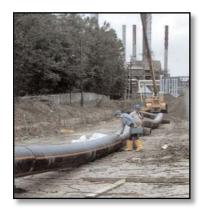
**DriscoPlex®** 4000/4100 Factory Mutual (FM) series – These HDPE PE4710 pipes and fittings are used for underground fire water protection systems for industrial and municipal applications. The pipe is manufactured with an optional single color stripe that are permanently extruded onto the pipe OD. The pipe has an ASTM D3350 Cell Classification of PE445574C and is available in pressure class 150 and 200 psi. The pipe conforms to ASTM F714, AWWA C906, ASTM D3035, AWWA C901, NSF 61 and FM 1613.
