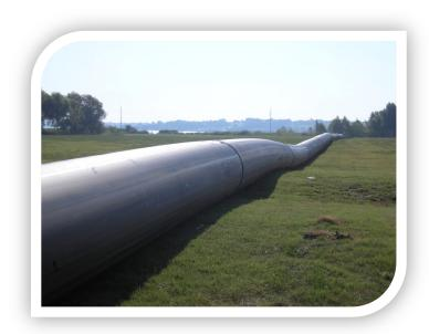
DRISCOPLEX® HDPE Pipe is available to meet your needs in compliance with ASTM D3035 or ASTM F714 product standards.
