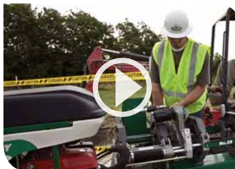
Using McElroy Equipment for In-Ditch Fusion Operations
