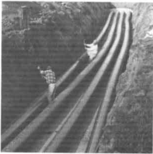
FIGURE 18 - Multiple Pipes in a Trench
