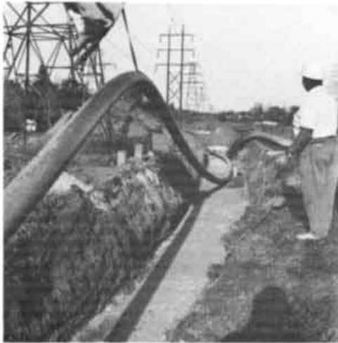
FIGURE 12 - Placing Pipe in the Trench
