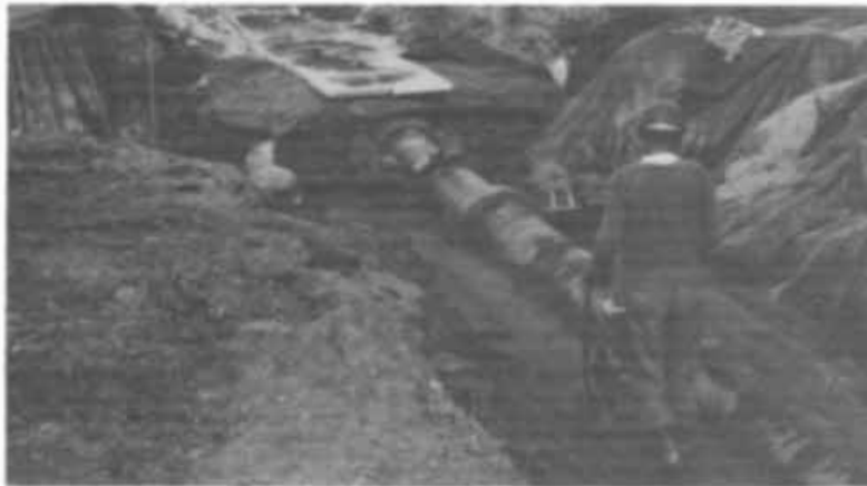
FIGURE 17 - Haunching Small Diameter Pipe
