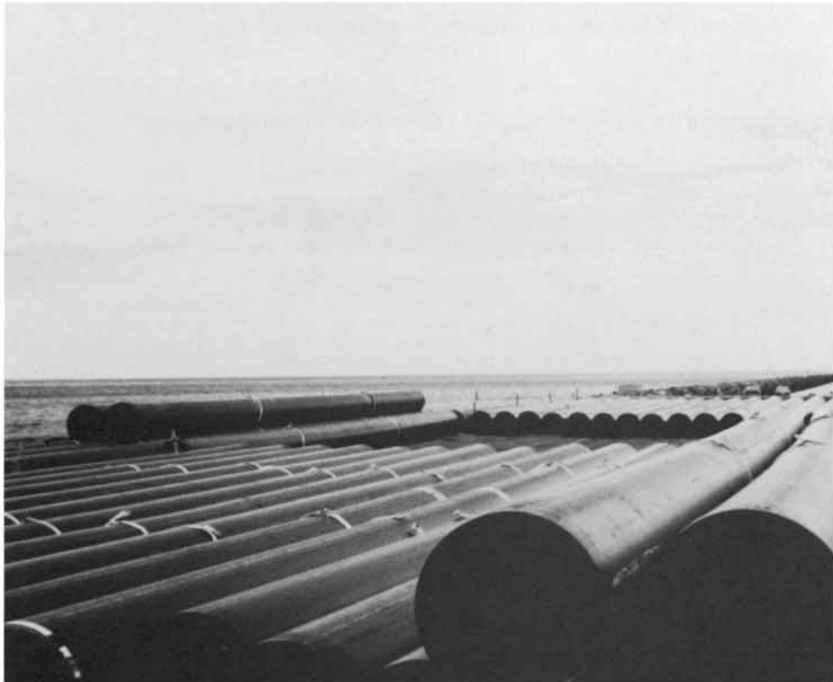
FIGURE 2 - On-Site Pipe Storage
