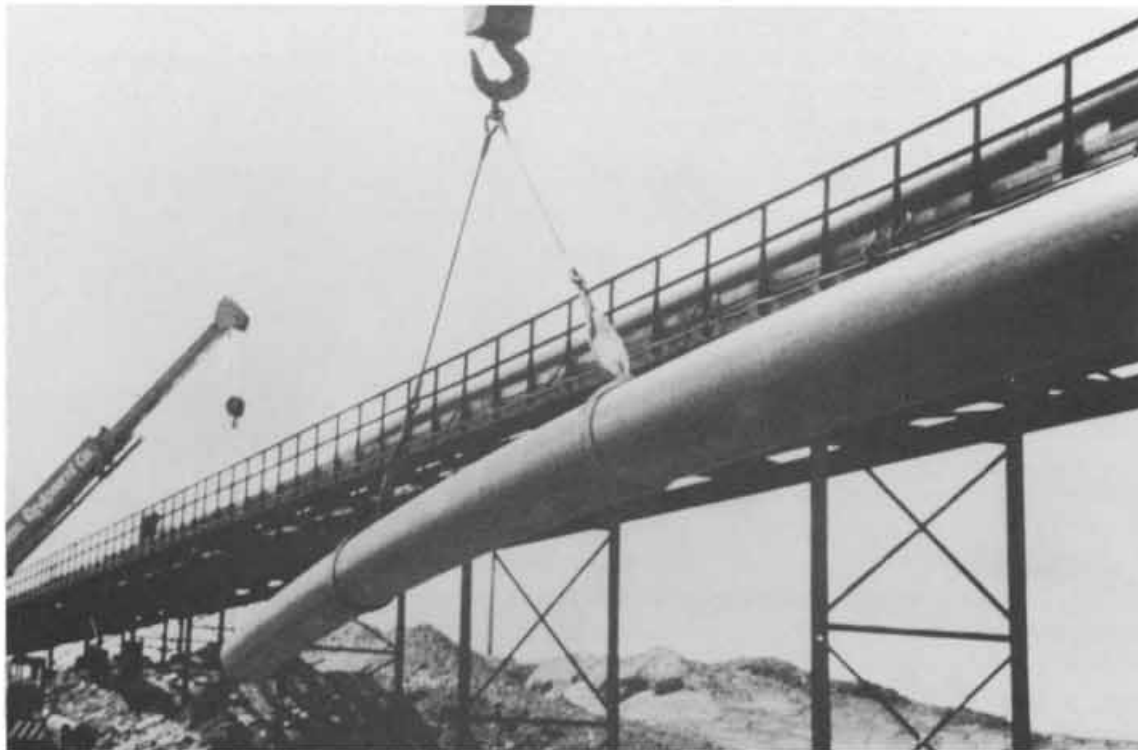
FIGURE 1 - Typical Handling Techniques
