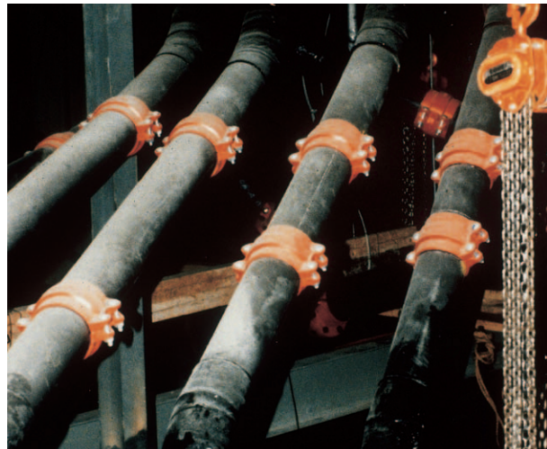
Polyethylene's abrasion resistance and chemical inertness were prime considerations in the decision to specify SCLAIRPIPE in this process pipe application.
